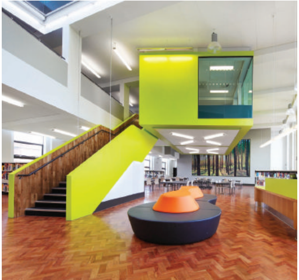
A new learning pod is suspended from existing beams to prevent extra loading on the floor.
