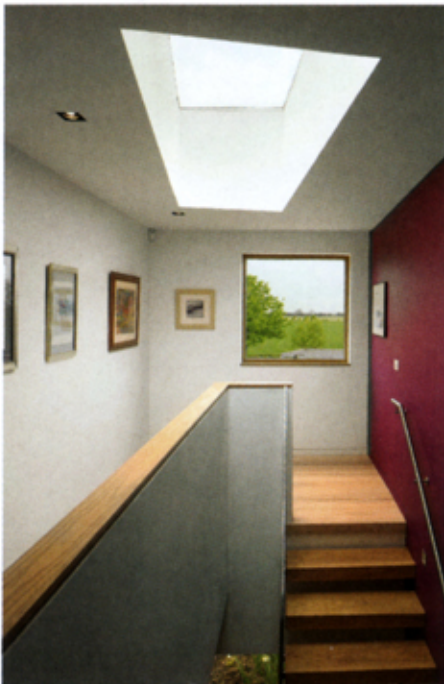
Below Stair treads cantilever from the double-height end wall
