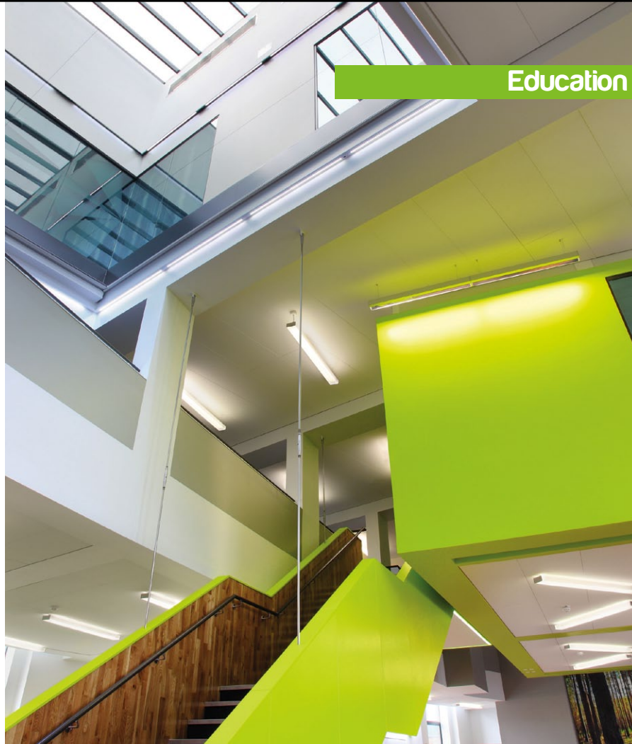
Further visual effects are gained by the insertion of a wide and deep lightwell piercing the two storeys above the learning centre and bringing additional natural light into the core of the building
